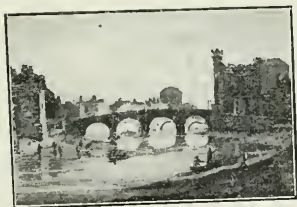
FIG. 49.—Barrack and Queen's Bridges. Petrie, 1819.
